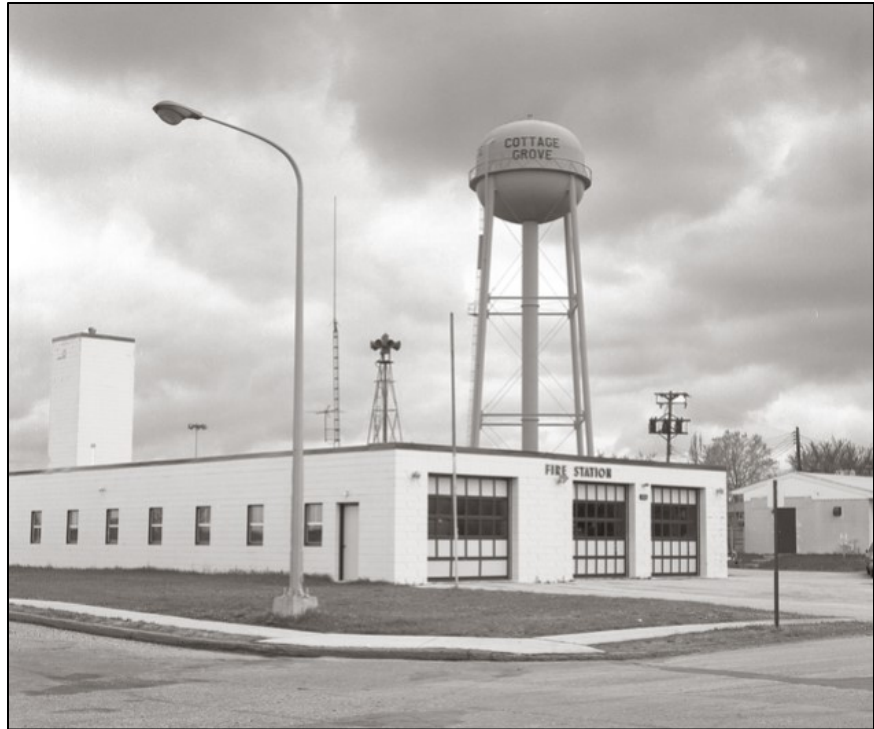
Figure 4.1. Grange Elevated Water Tower and Fire Station No. 1, looking south from Grange Boulevard, 1983. Image courtesy of MNHS.
