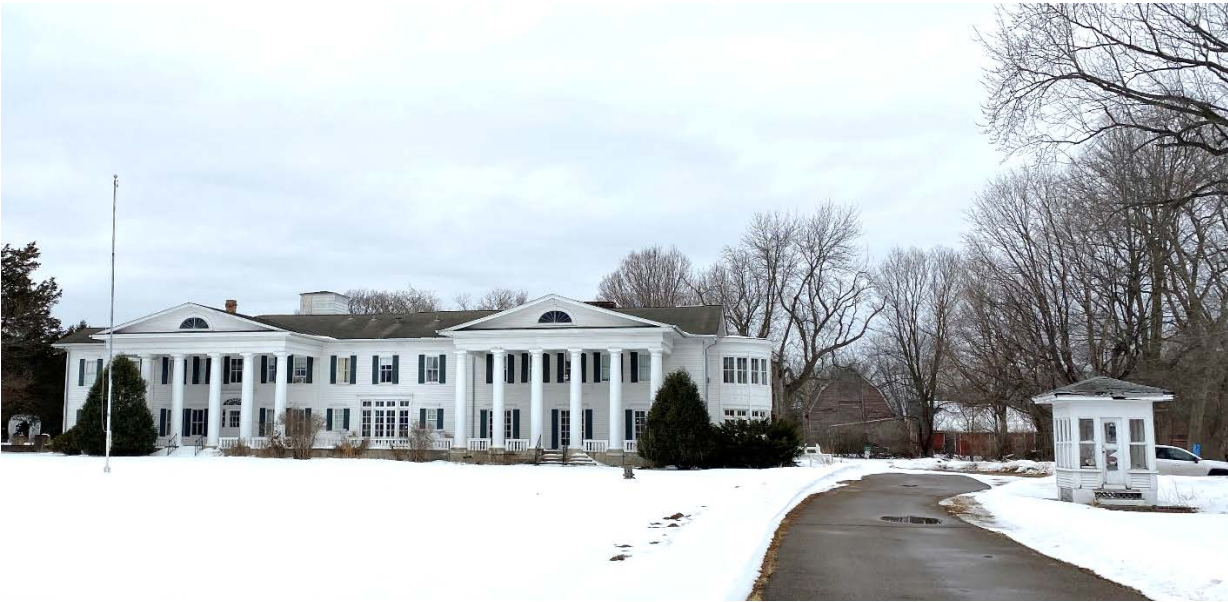
Figure 1: View of the Cordenio Severance House and Valet Shelter, looking west.
