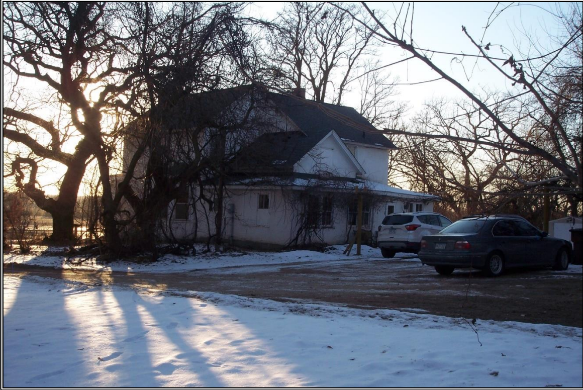
Looking SW at rear and east sides of house on property
