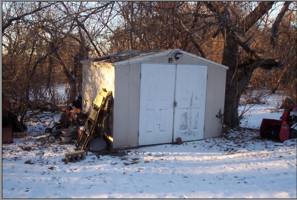
Westerly view of metal storage shed on concrete slab located about 20' NW of house
