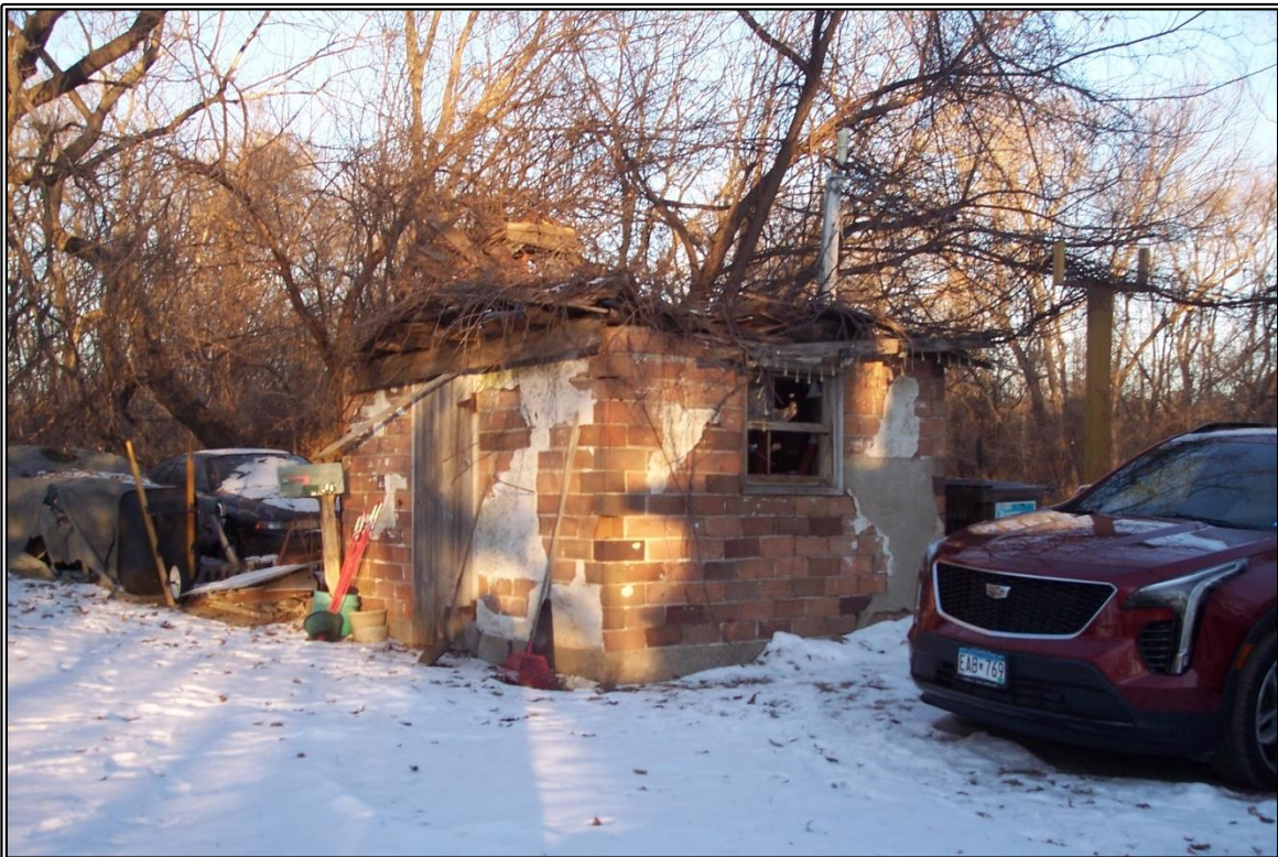
Northerly view of old pump house (no longer in use) located about 30' NE of house
