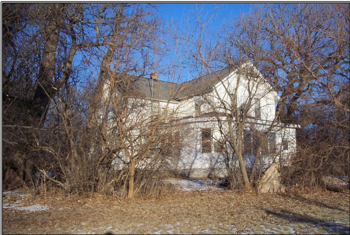
Looking NE at front (south) and west sides of house on property
