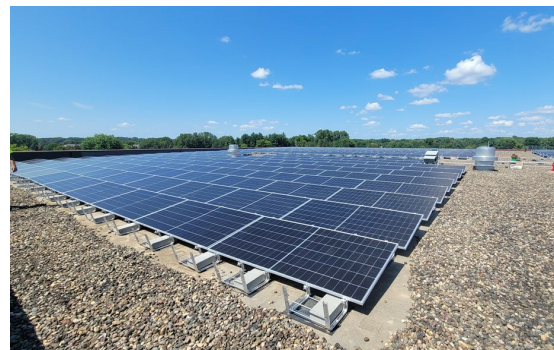
Cottage Grove Ice Arena
