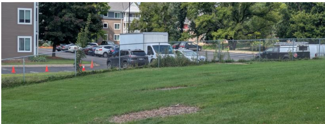
Existing Chain Link Fence on West Side
