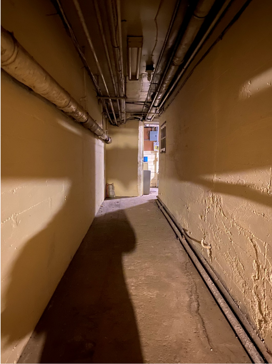
Photo 23. View of tunnel between Wing B and Wing A at lower level of Severance House, looking east.
