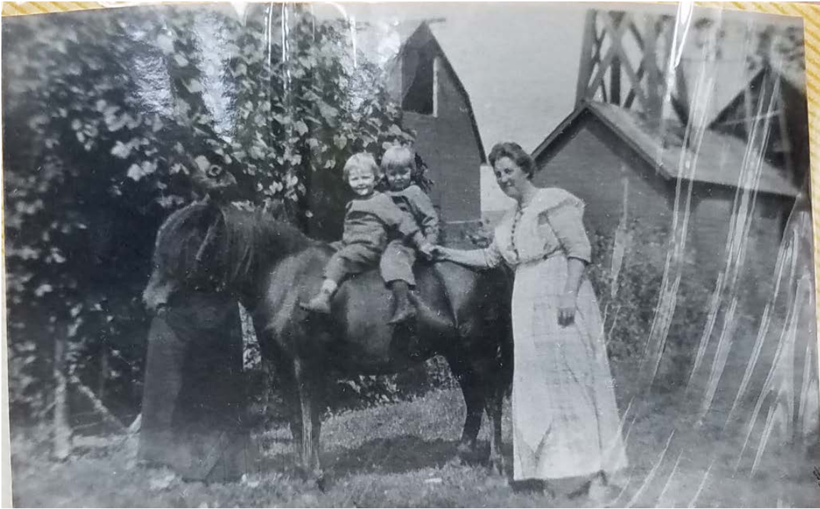
Figure M. View of east elevation of barn, looking northwest, likely 1925 or earlier. Photograph courtesy of the City of Cottage Grove.
