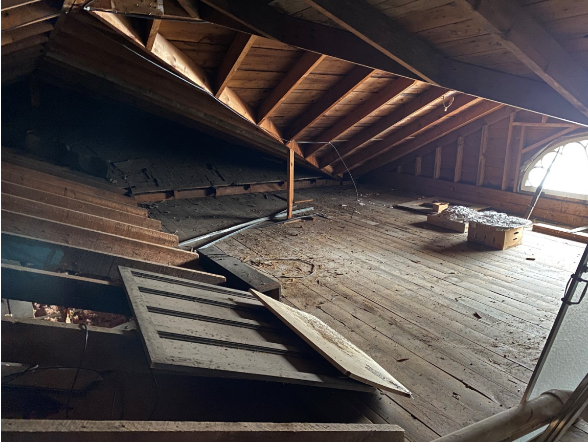
Photo 49. View of attic at Severance House (Wing A), looking southwest.
