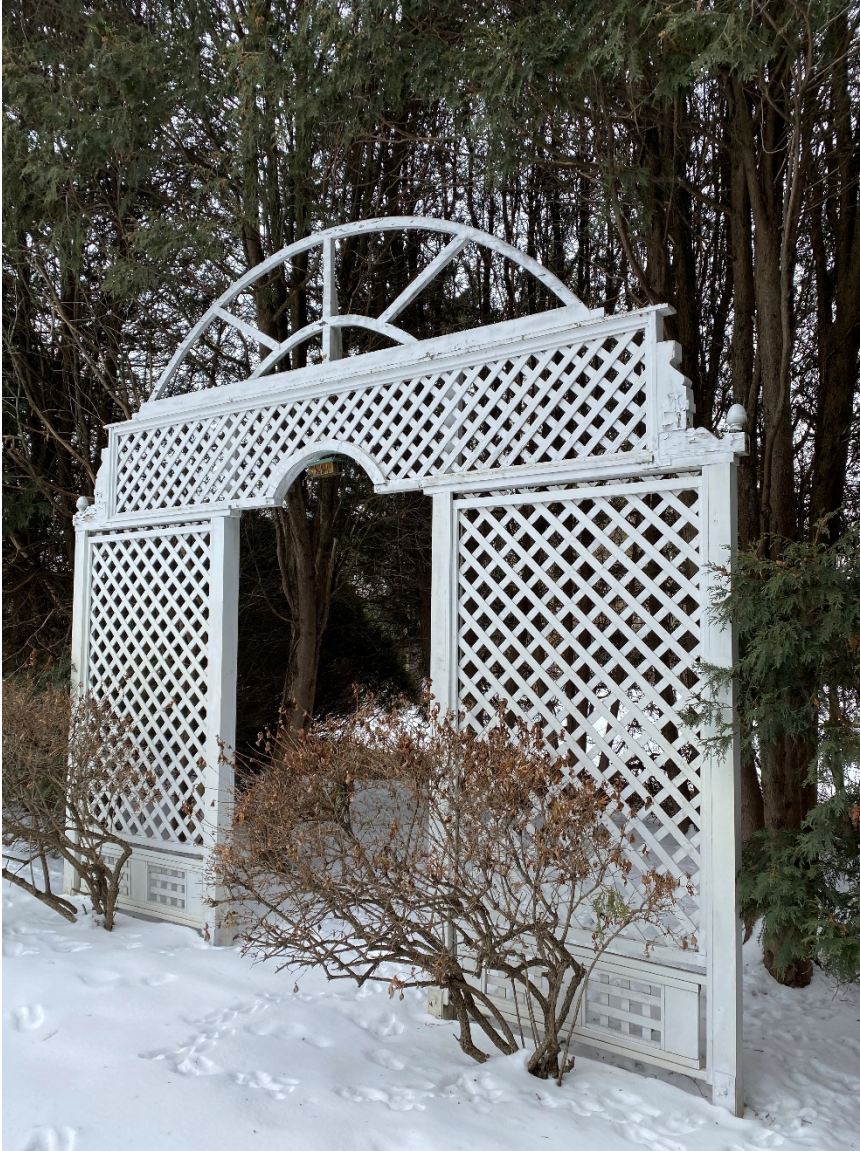
Photo 61. View of trellis, looking southeast.
