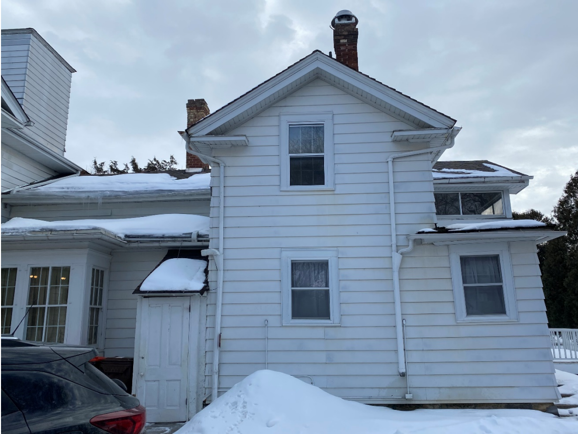
Photo 13. View of north elevation of Severance House (Wing B), looking south.
