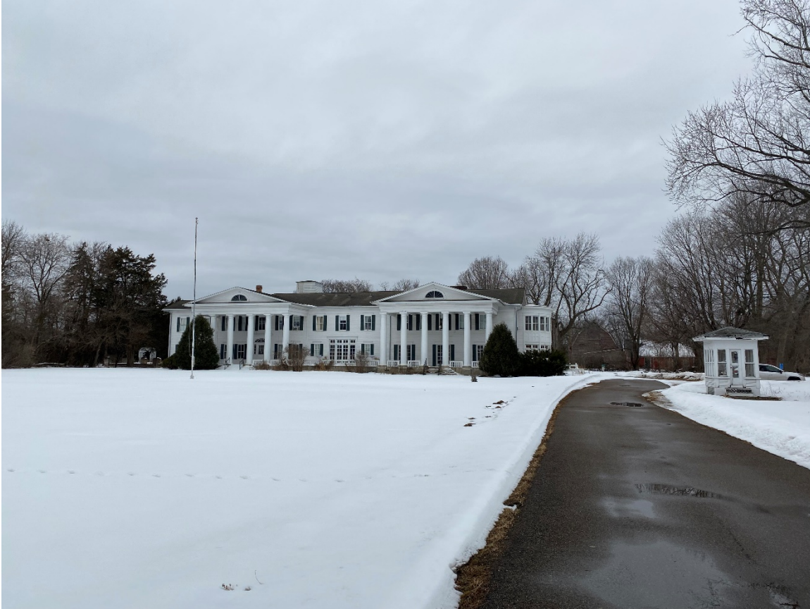
Photo 3. View of east elevation of Severance House (Wing A), looking west.
