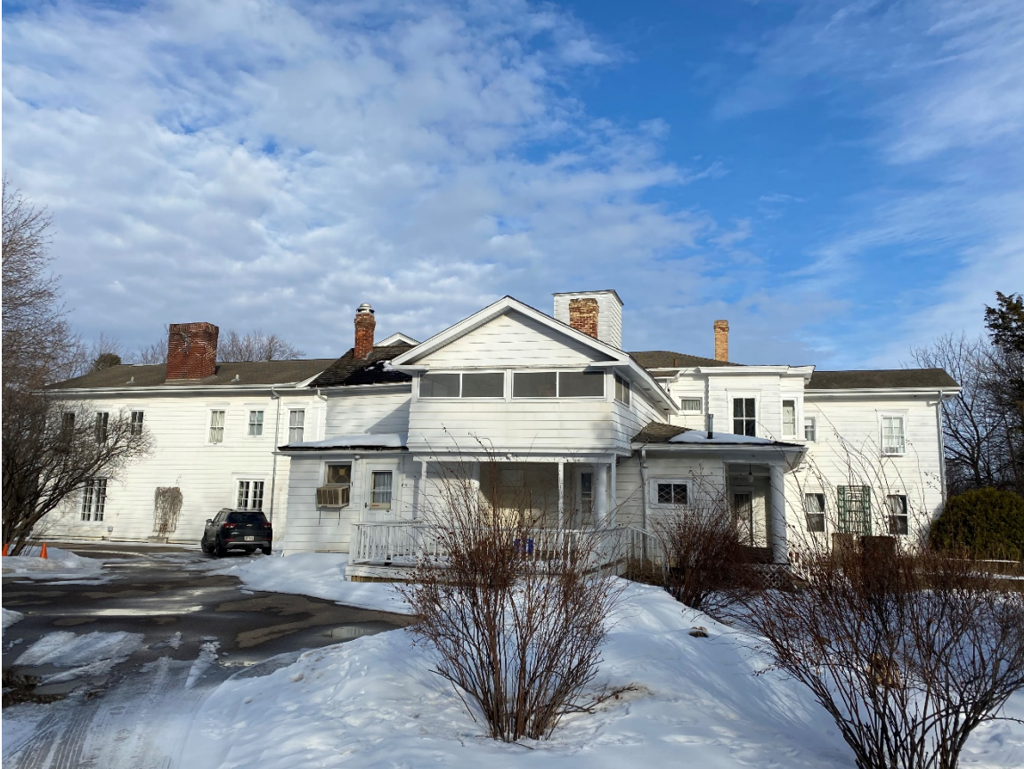
Photo 11. View of west elevation of Severance House, looking east.
