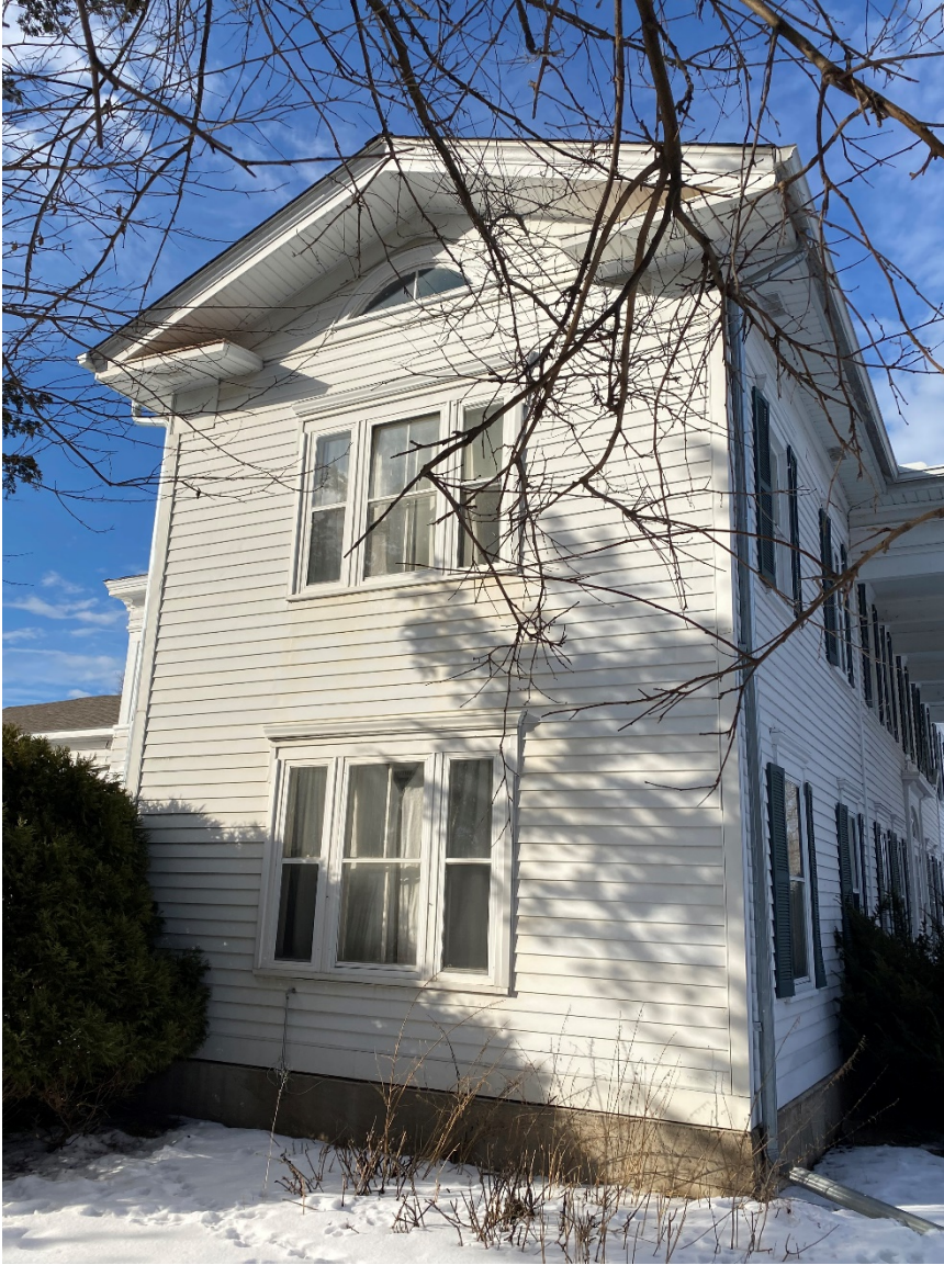
Photo 17. View of south elevation of Severance House (Wing A), looking northwest.
