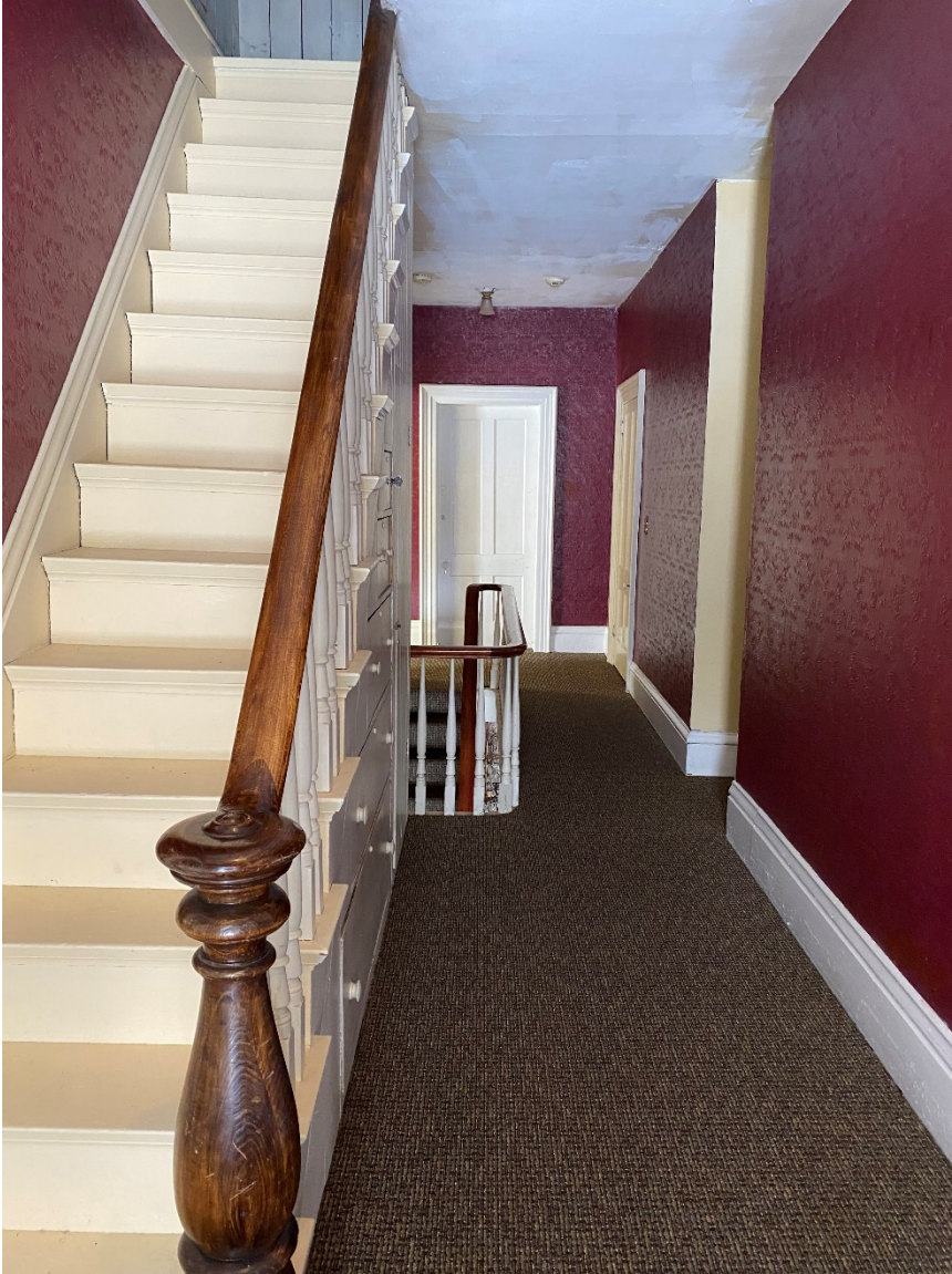
Photo 41. View of second-level corridor at Severance House, looking west.
