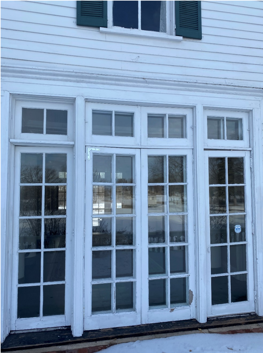
Photo 20. View of central entrance on east elevation of Severance House, looking west.
