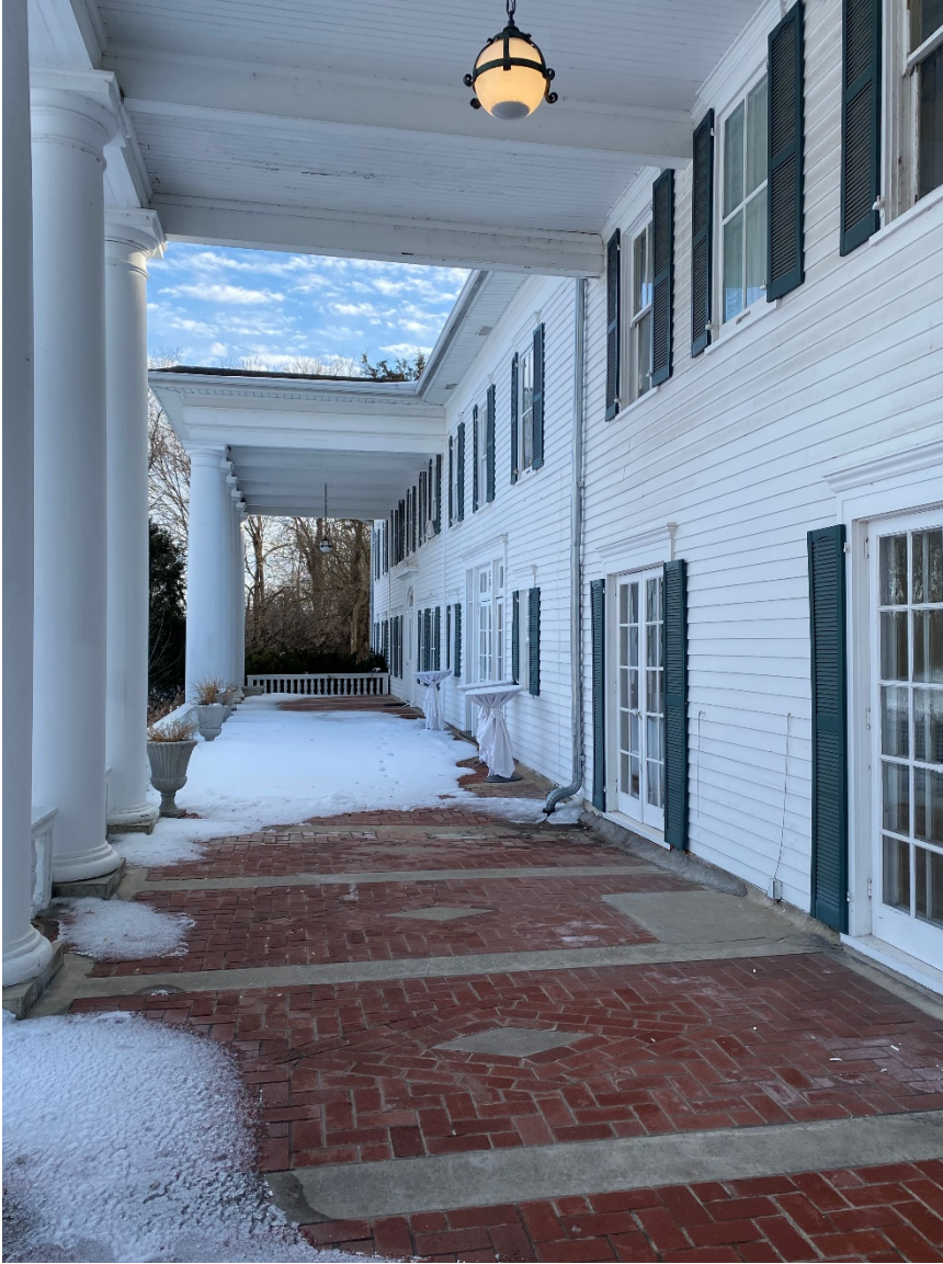
Photo 19. View of east elevation of Severance House, looking southwest.
