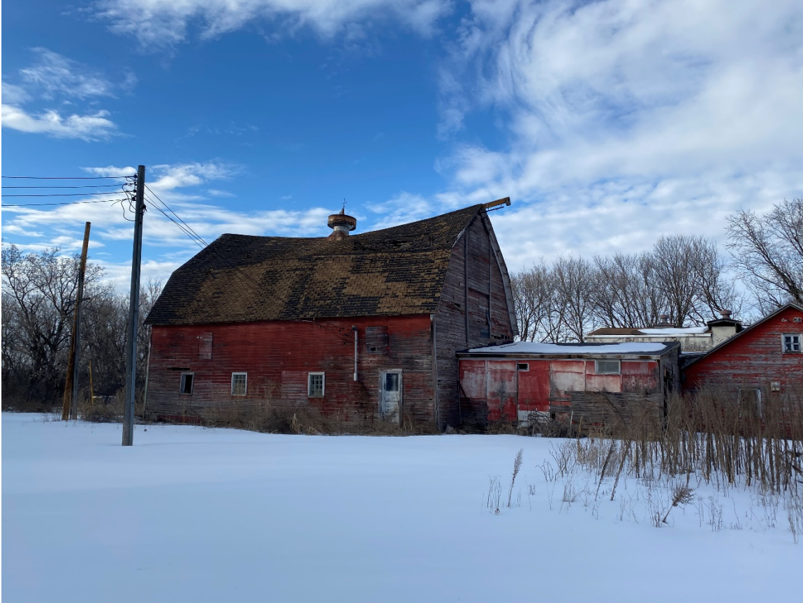
Photo 52. View of south and east elevations of the barn, looking northwest.
