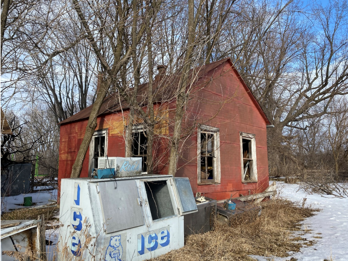
Photo 57. View of west and south elevations of shed #1, looking northeast.
