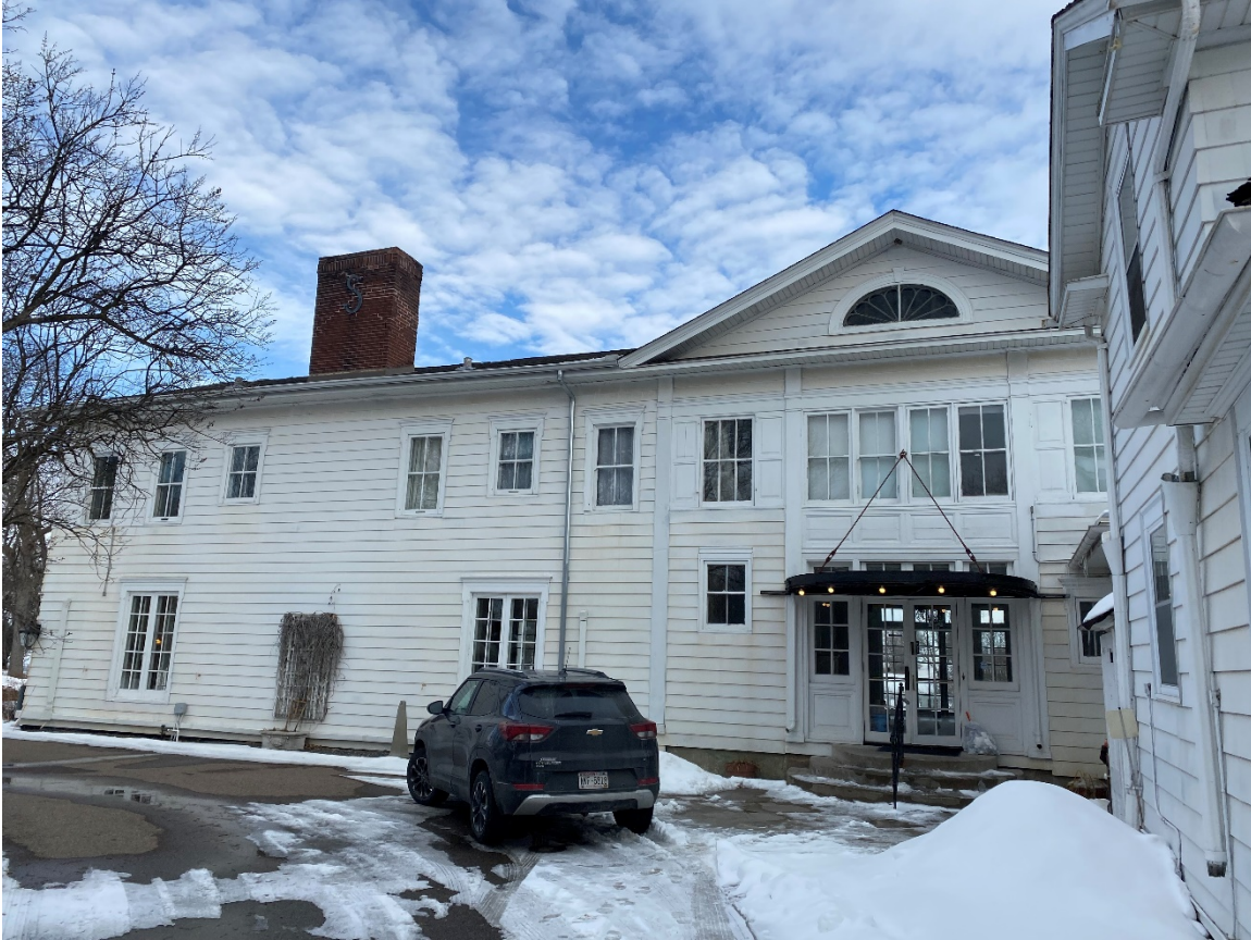
Photo 12. View of west elevation of Severance House (Wing A), looking east.
