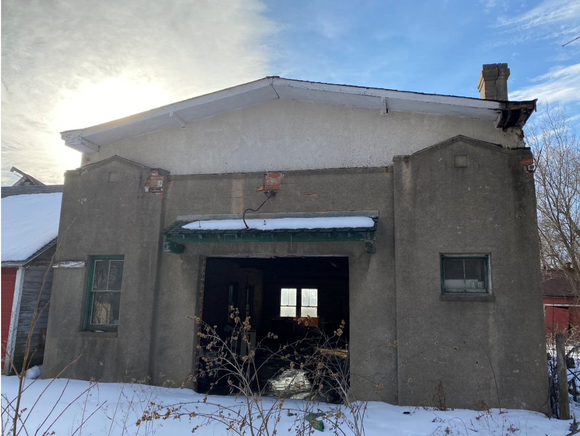
Photo 53. View of east elevation of garage, looking west.
