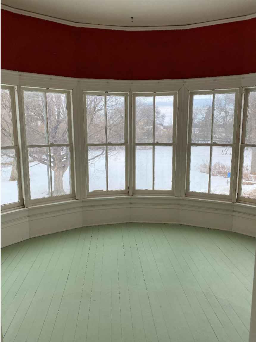
Photo 38. View of second-level sunroom at Severance House (Wing A), looking north.
