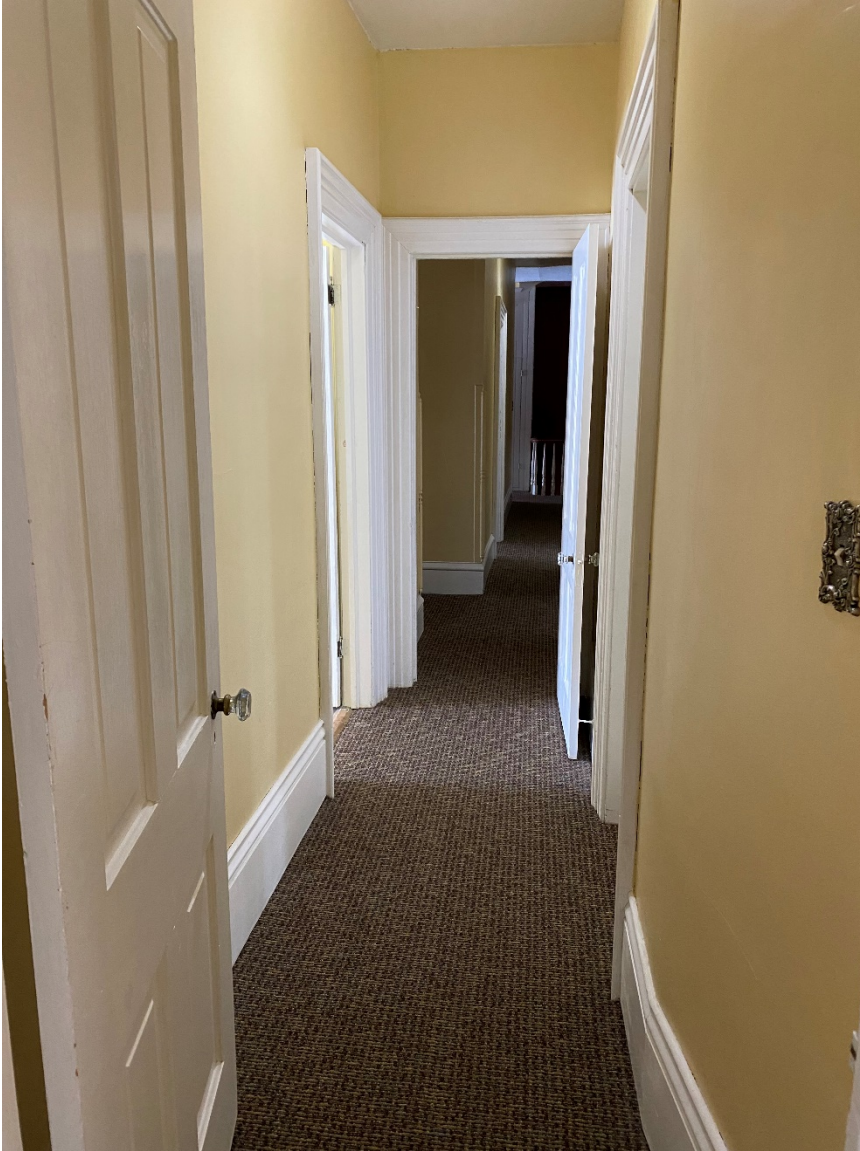
Photo 40. View of second-level corridor at Severance House (Wing A), looking south.
