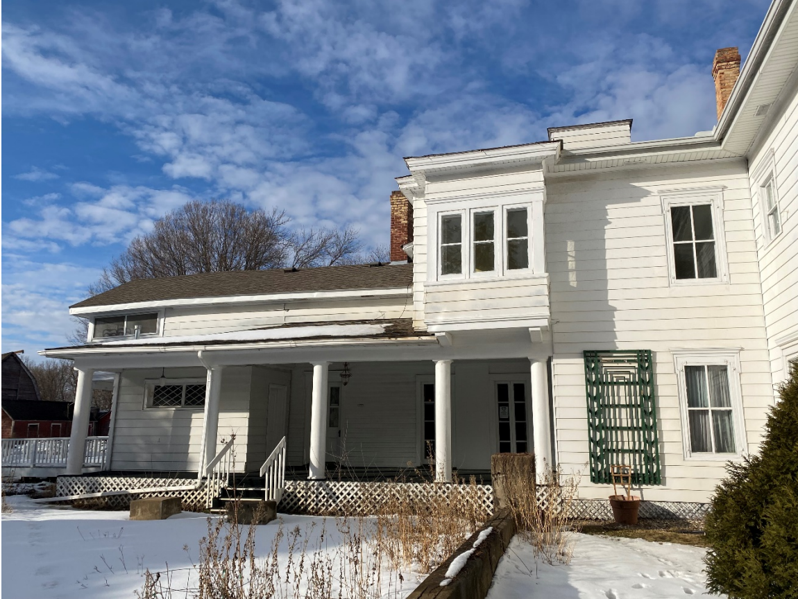
Photo 15. View of south elevation of Severance House (Wing B), looking north.
