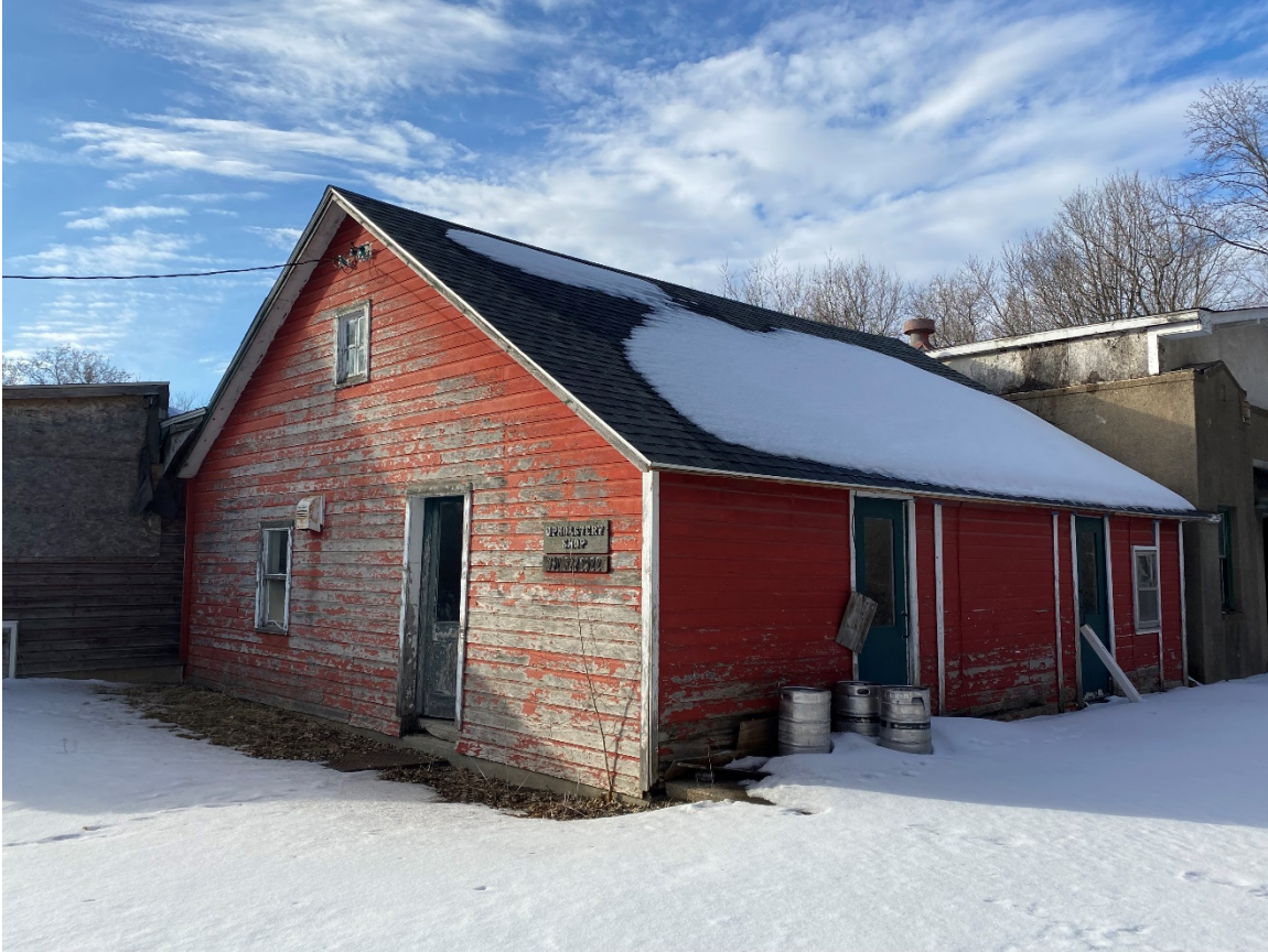
Photo 55. View of south and east elevations of upholstery shop, looking northwest.
