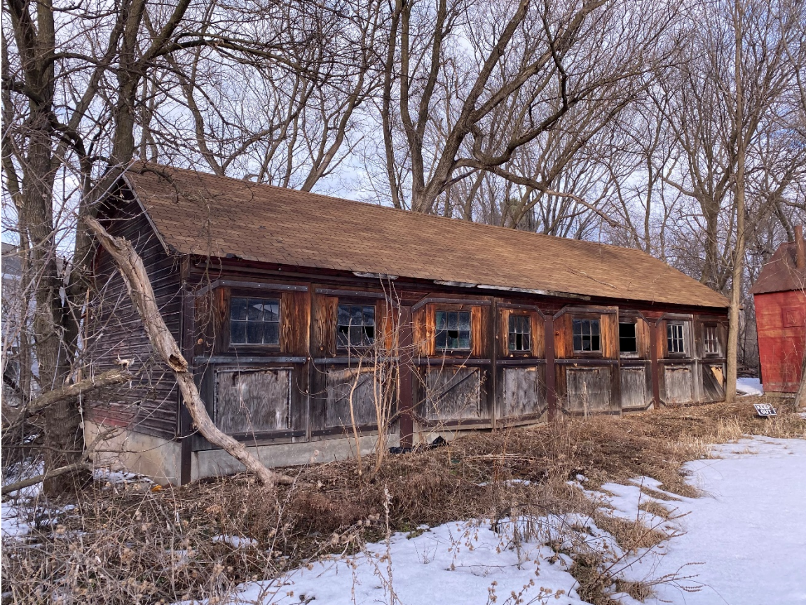
Photo 58. View of west and south elevations of shed #2, looking northeast.
