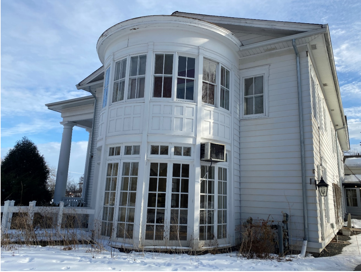
Photo 10. View of north elevation of Severance House (Wing A), looking southeast.
