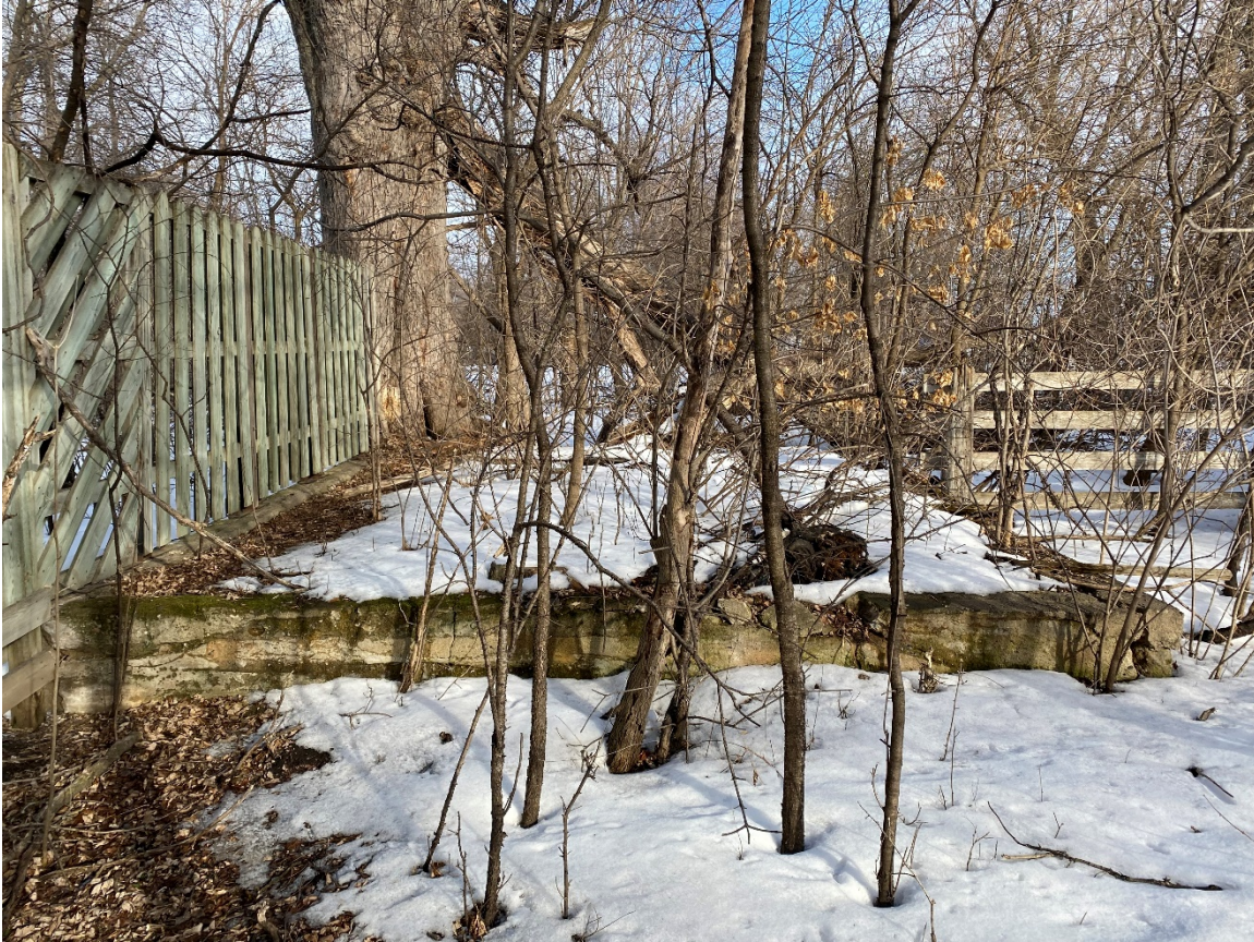
Photo 60. View of building foundation, looking east.
