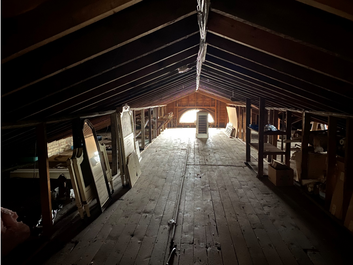
Photo 48. View of attic at Severance House (Wing A), looking north.
