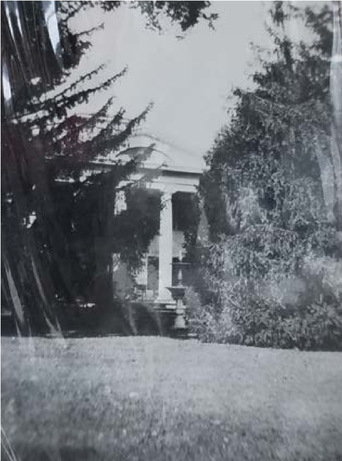
Figure E. View of east lawn and east elevation of Severance House, looking northwest, pre-1917. Photograph courtesy of the City of Cottage Grove.
