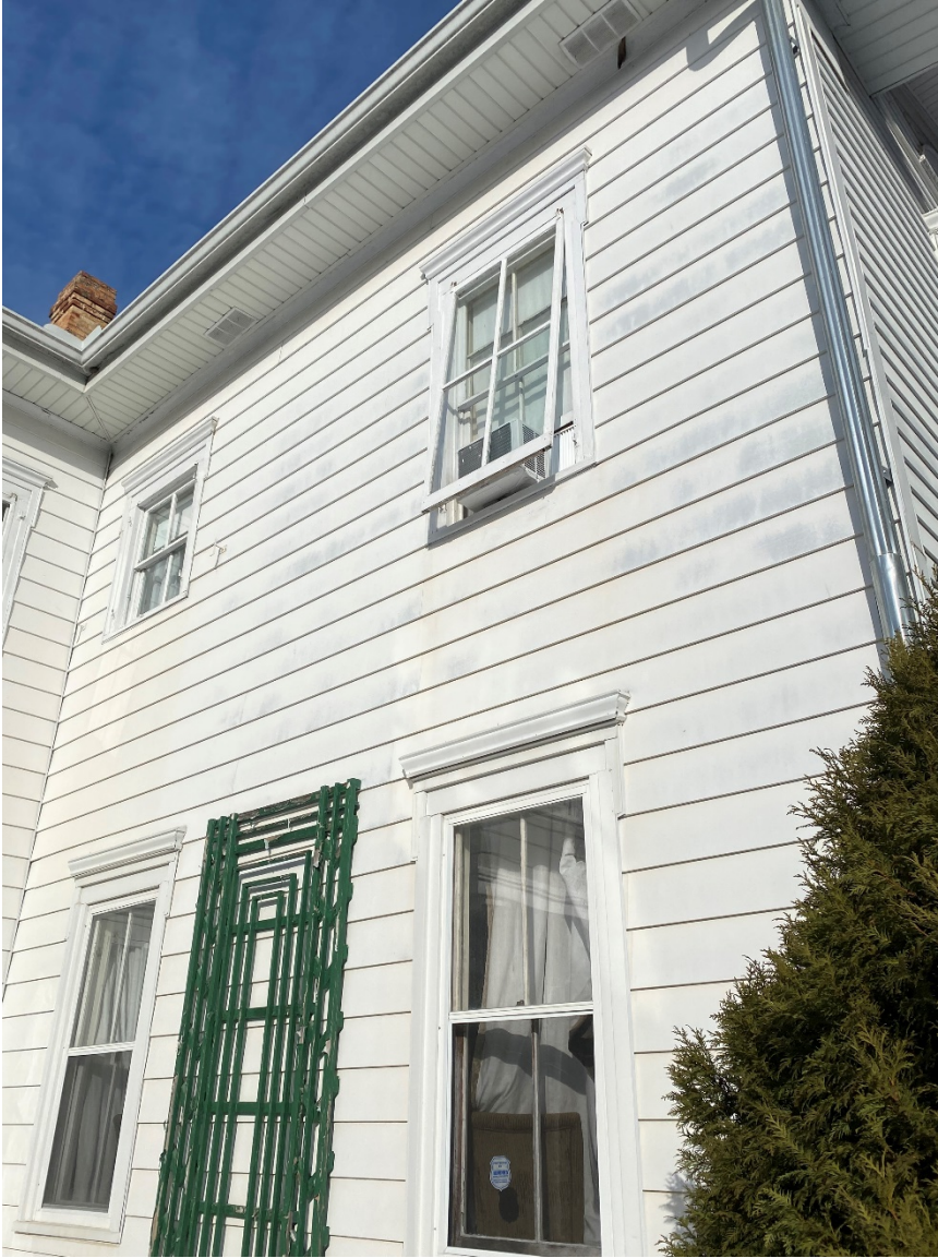
Photo 16. View of west elevation of Severance House (Wing A), looking northeast.
