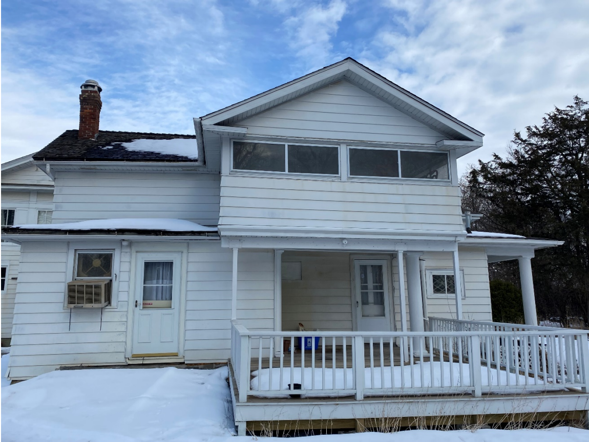
Photo 14. View of west elevation of Severance House (Wing B), looking east.
