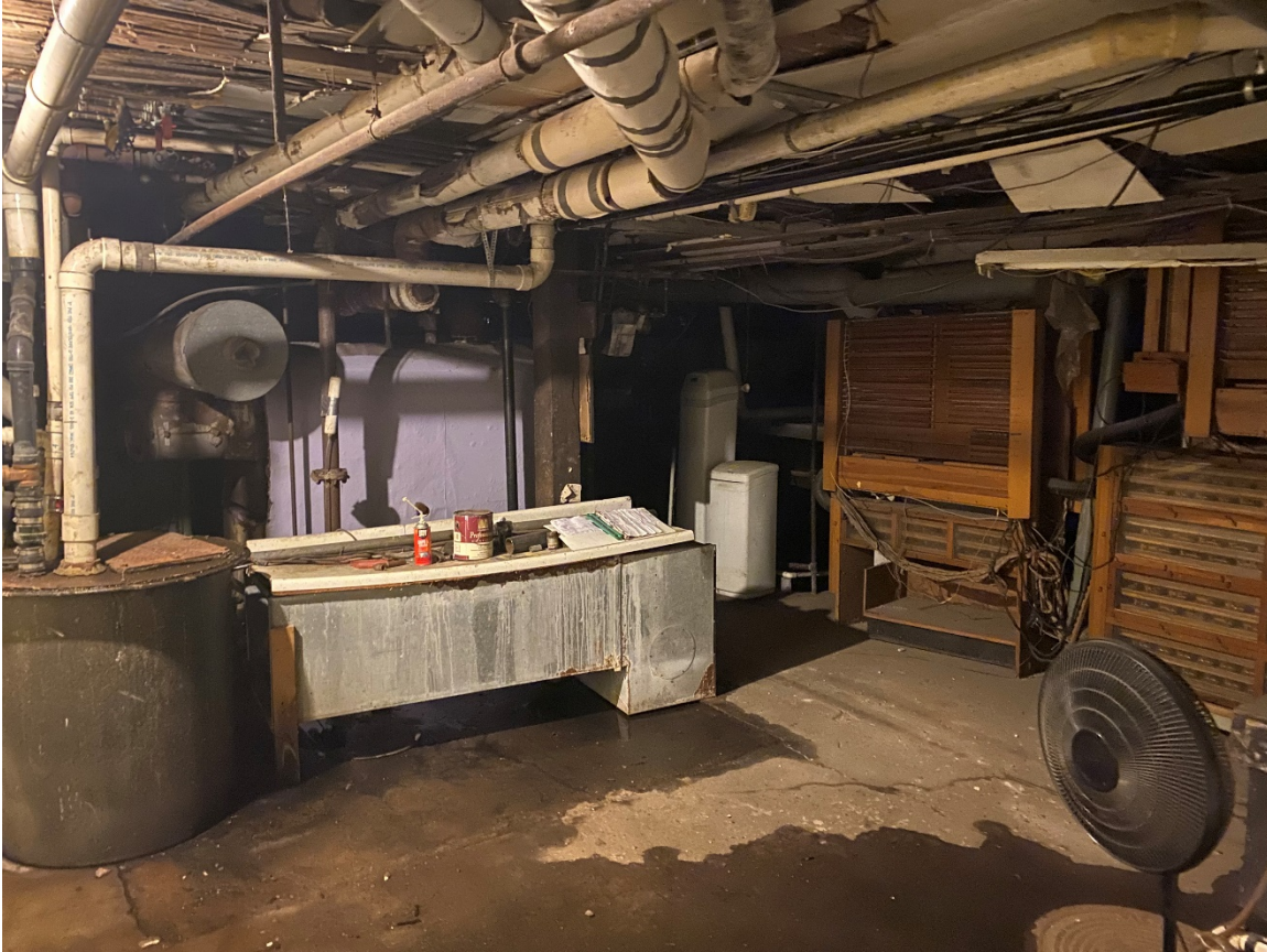
Photo 24. View of lower level of Severance House (Wing A), looking northeast.
