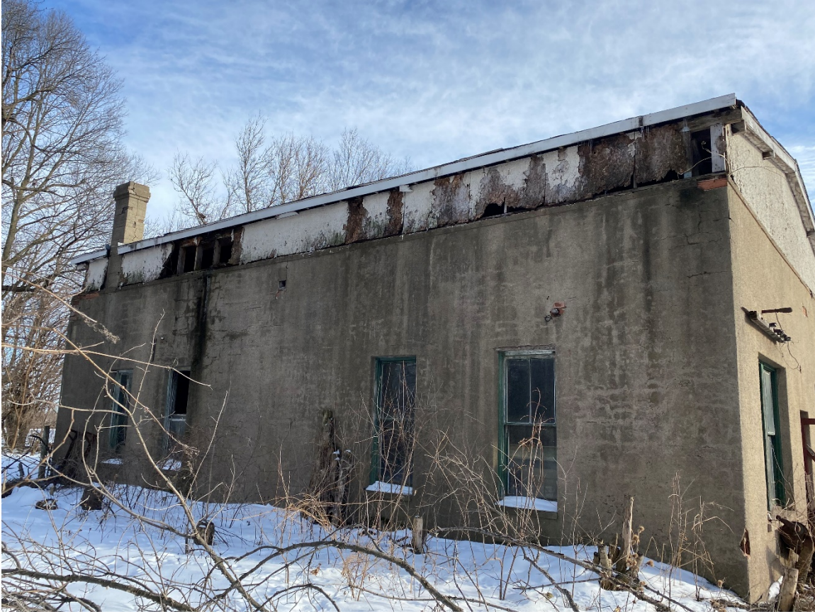
Photo 54. View of north elevation of garage, looking southeast.
