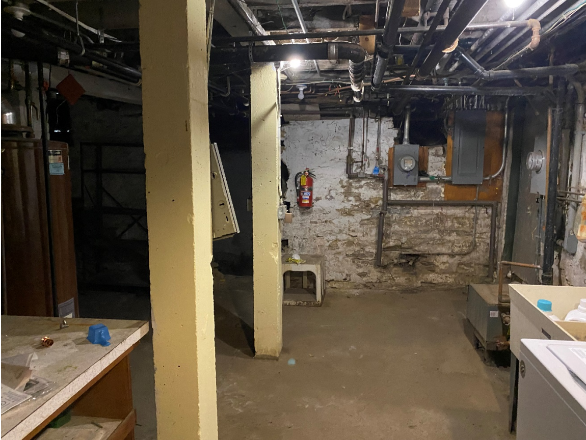
Photo 21. View of lower level of Severance House (Wing B), looking south.
