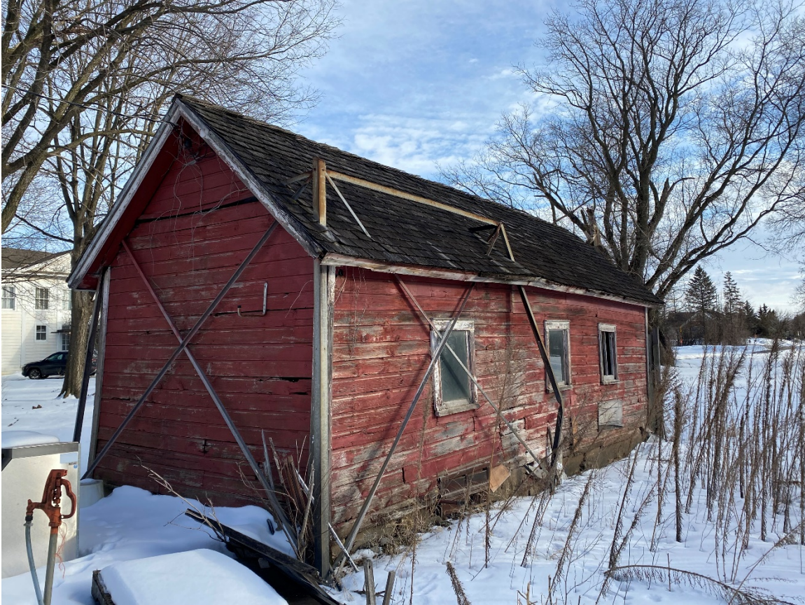
Photo 56. View of north and west elevations of chicken coop, looking southeast.
