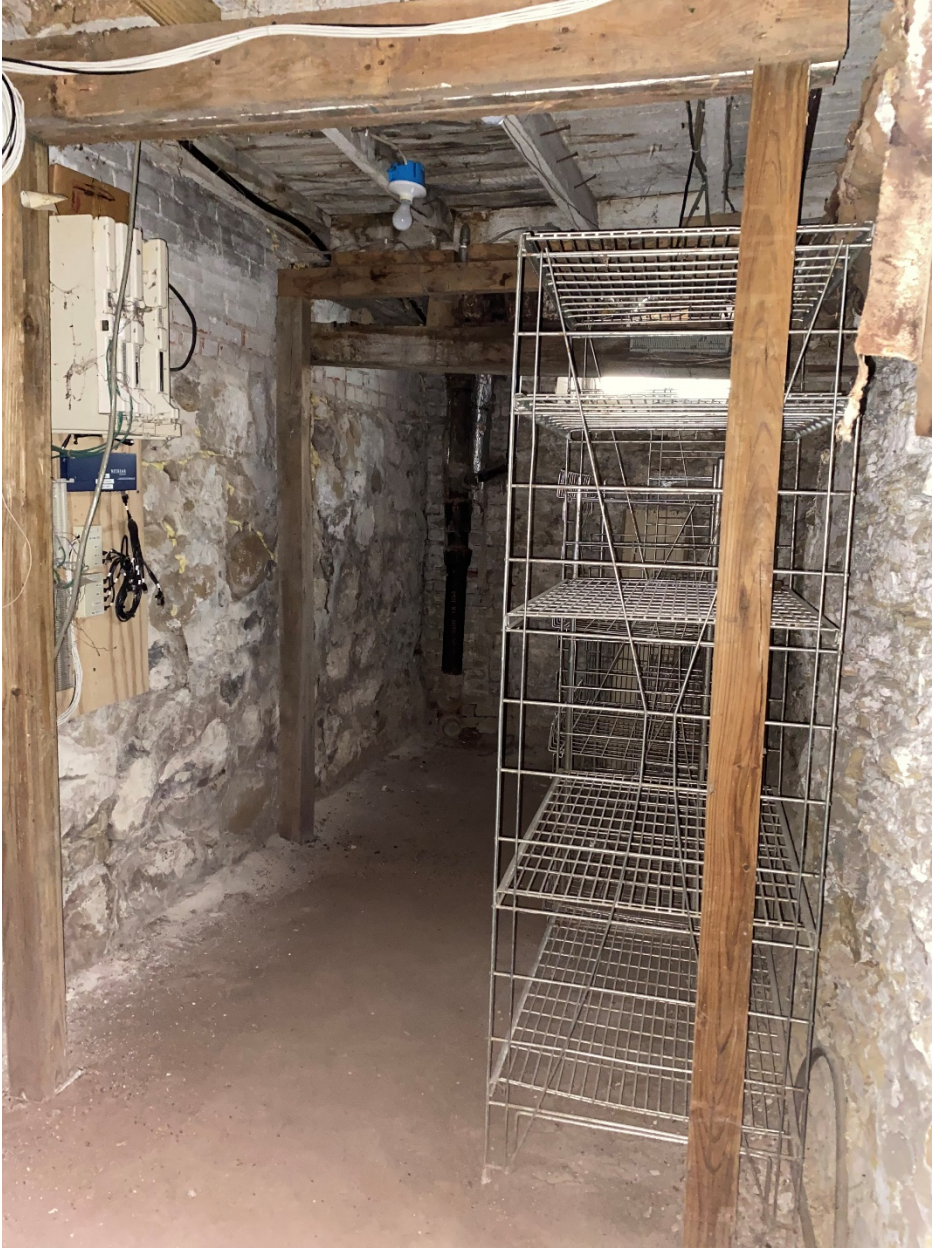
Photo 22. View of lower level of Severance House (Wing B), looking south.
