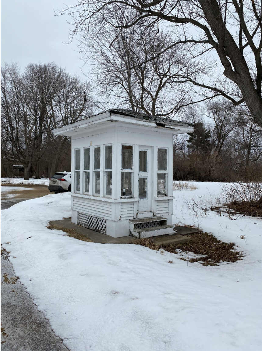
Photo 59. View of south and east elevations of valet shelter, looking northwest.
