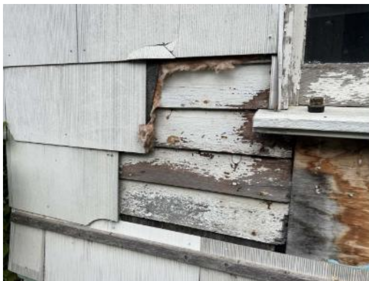
Original Clapboard Siding Underneath Asbestos Siding
