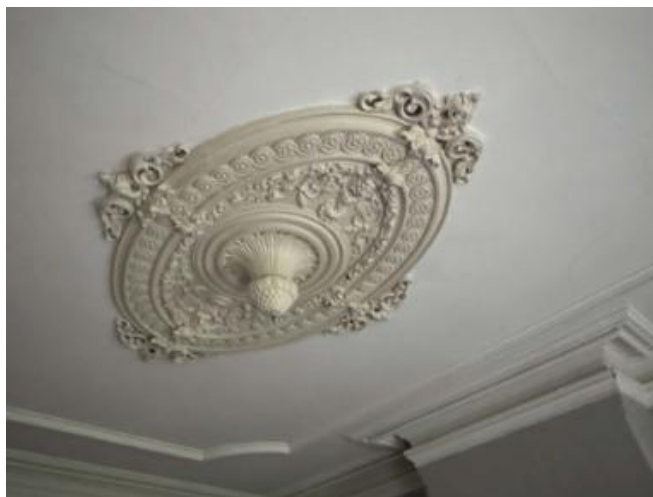
Interior Feature to Remain
