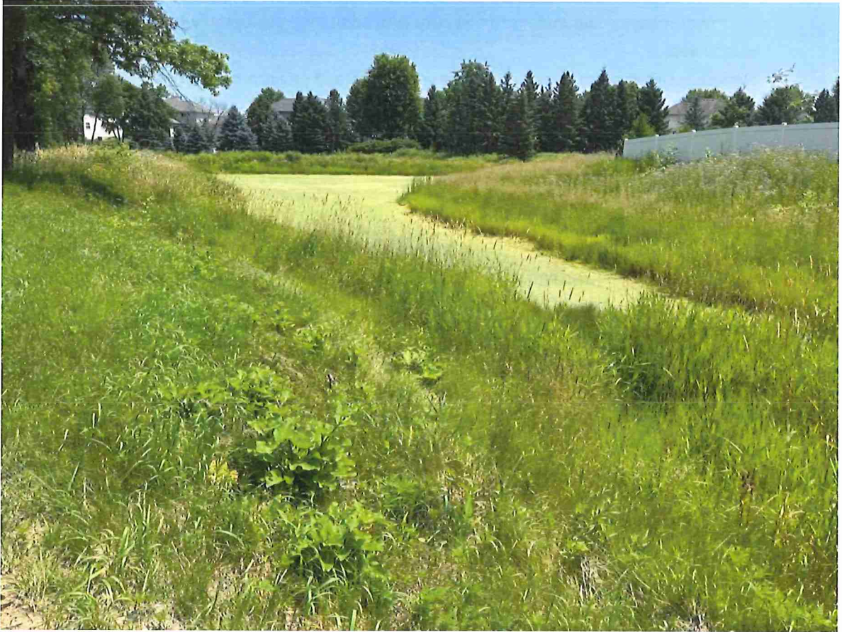
Figure 16. Stormwater Retention Pond at Still Ponds
