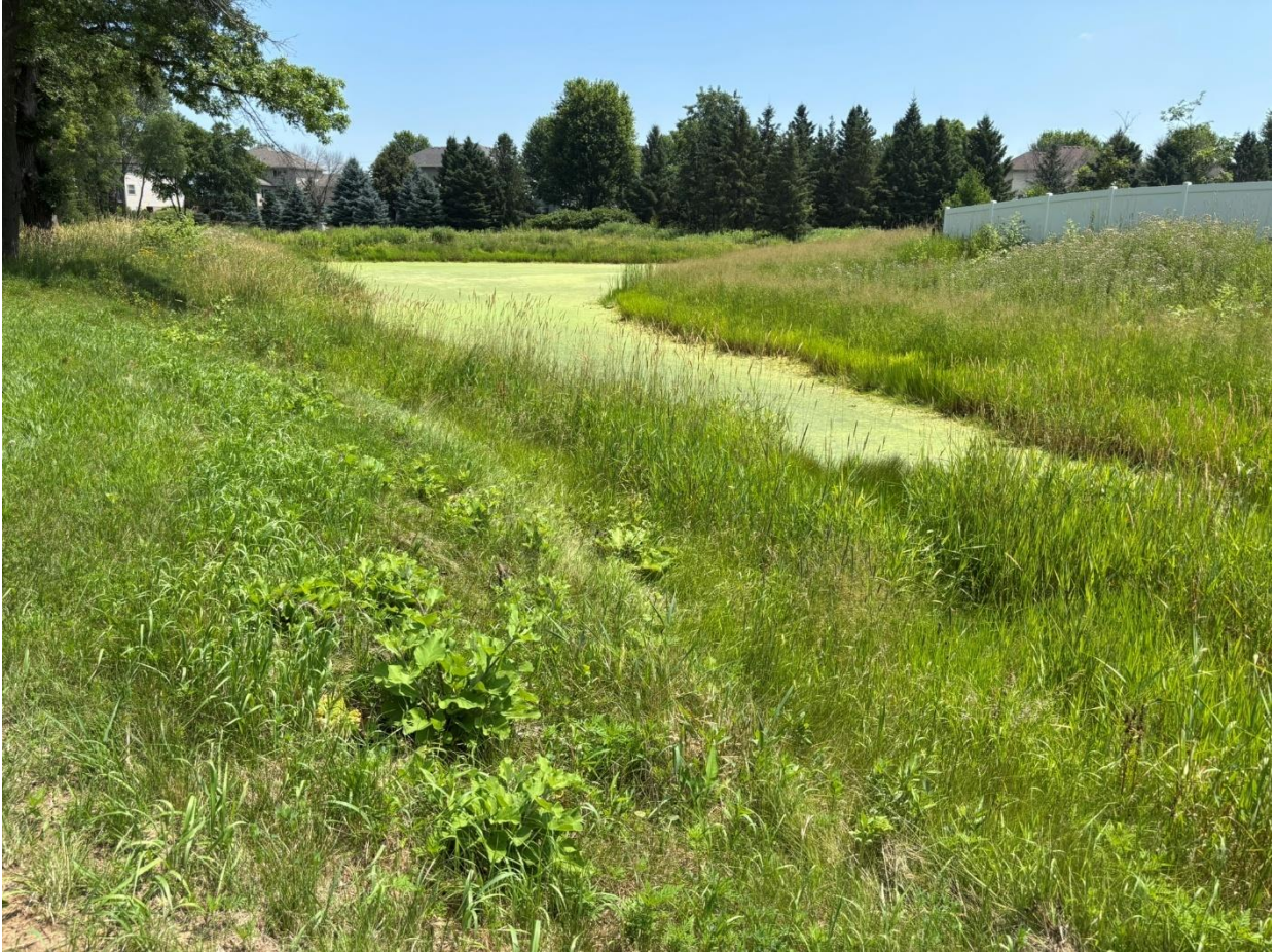
Figure 16. Stormwater Retention Pond at Still Ponds
