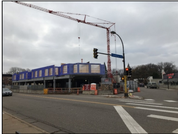
The Lorient: currently under construction
