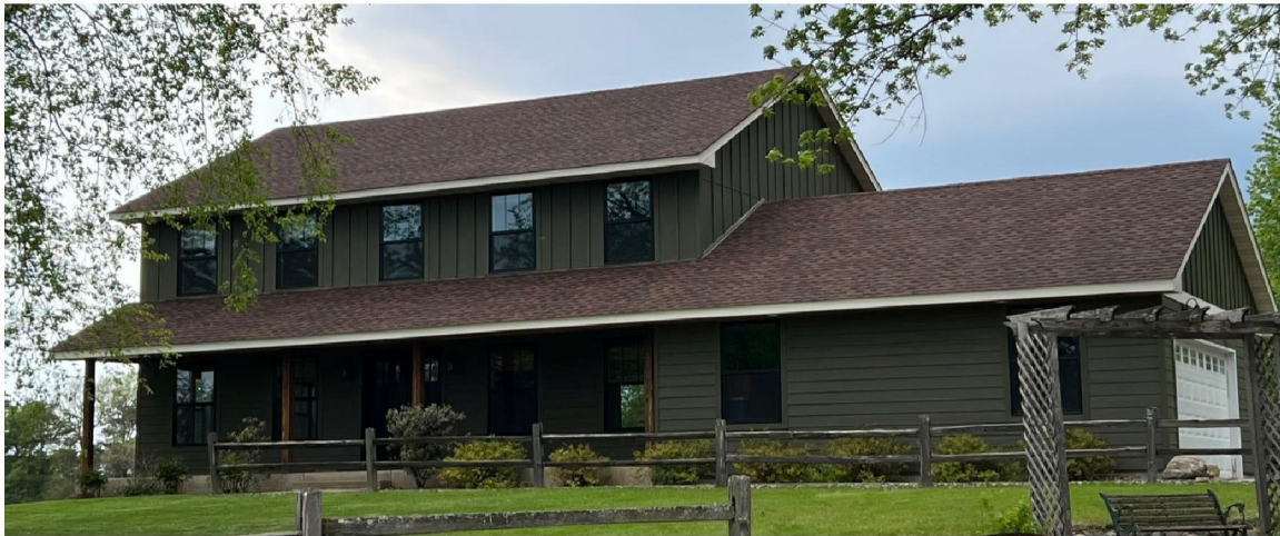
Photo of the house to be moved
