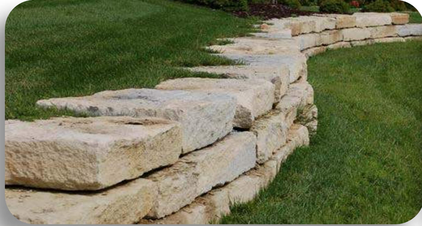
LIMESTONE RETAINING WALL
