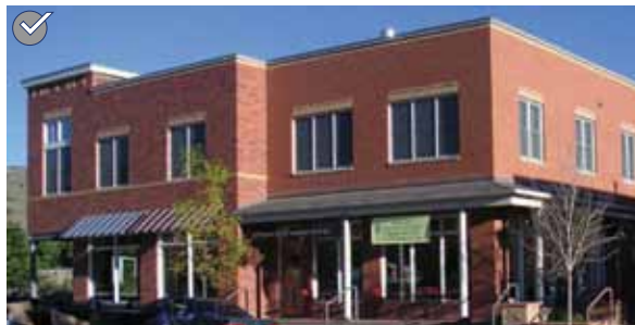
For larger buildings, new construction should incorporate design features that break down the mass into modules that suggest the underlying historic height, width and lot pattern.
