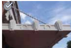
Preserve significant stylistic and character-defining features, such as this canopy.
