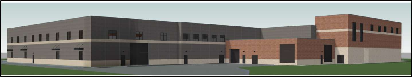
Water Treatment Plant – North Elevation (Facing the Central Fire Station)
