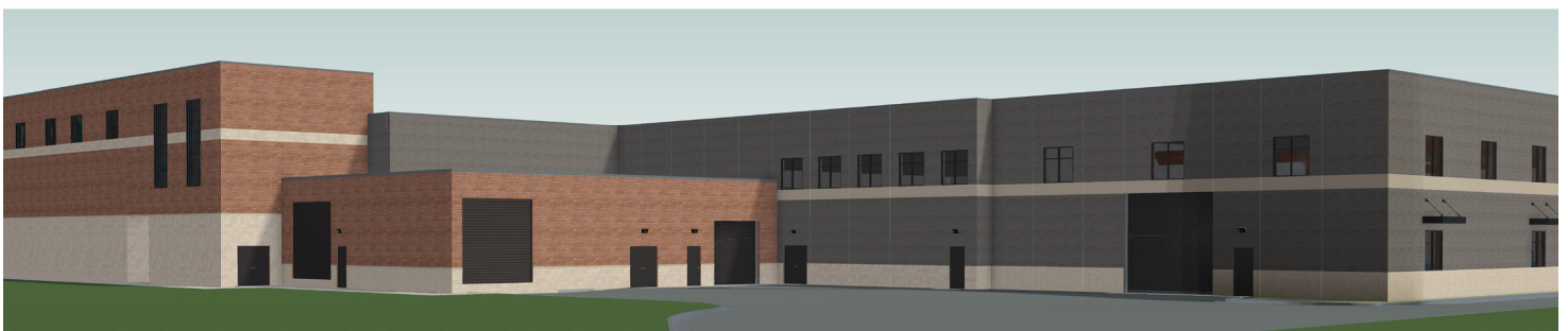
Intermediate Zone Treatment Plant
