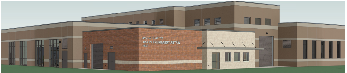
Low Zone Water Treatment Plant
