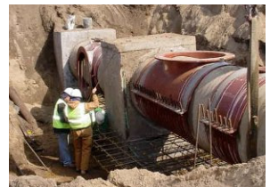
Construction of the regional sanitary sewer interceptor in 2004 opened up the East Ravine area for staged development.
