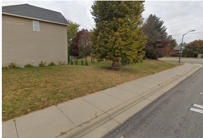
Figure 4: Back of curb sidewalk on the west side of Meadow Grass Avenue, northbound exiting the Pine Summit Development.
