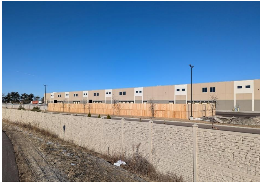
Existing Site Conditions
